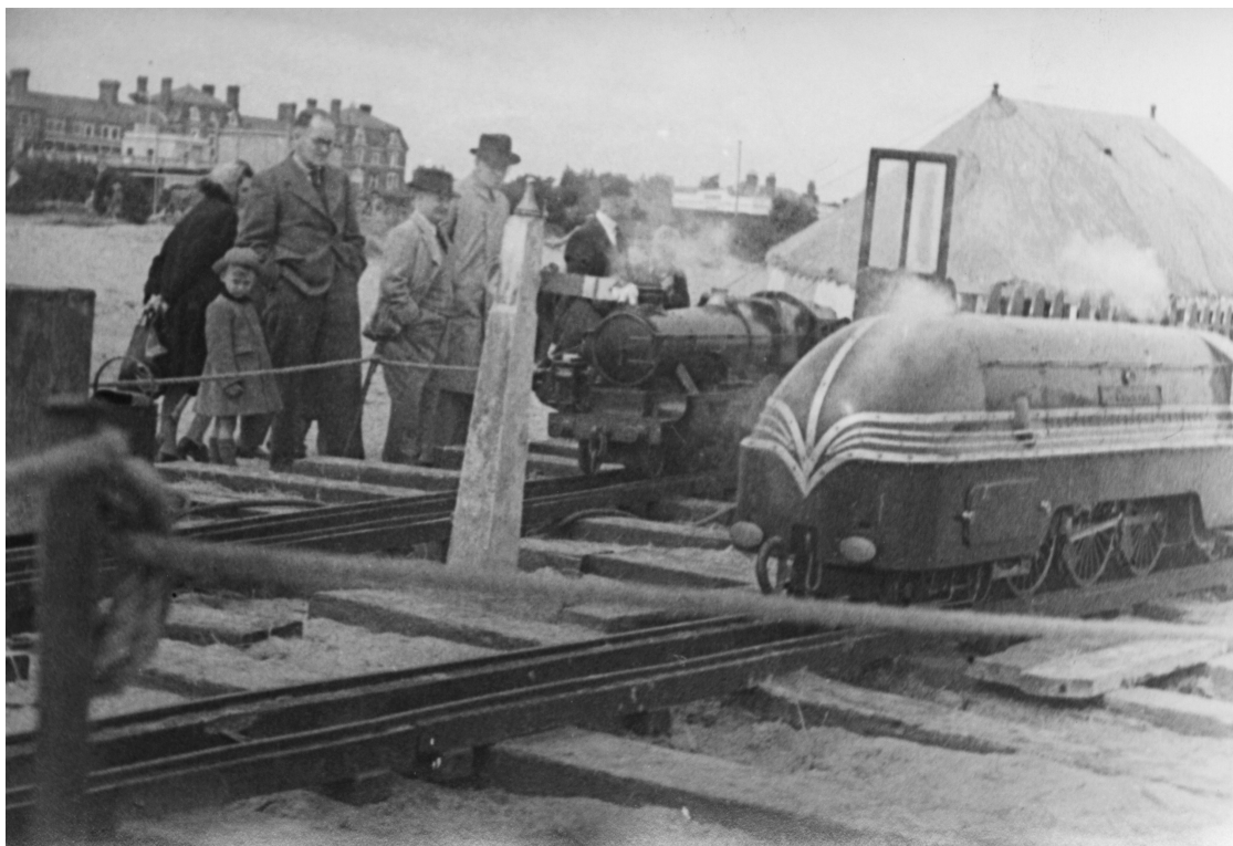
Photographs of the "tour" railways are rare. This view of the line on the Beach at Skegness in August 1946 is full of interest. No.1944 and "Coronation" rest in the station. Note the unusual track and the mainline railway sleepers, which have been utilised to support the track on the dunes. The marquee housing the model exhibition is behind the locomotives.
