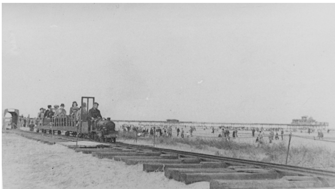
Another view of the railway on the dunes at Skegness - note the pier, much of which was lost in 1978. No.1944 has just left the tunnel and is passing over a level crossing. Note the normal rails used here, but still laid on mainline sleepers and extra pieces of wood.
