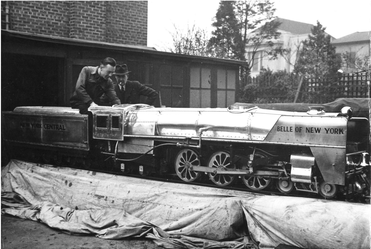
"Belle of New York" Here we see the newly completed locomotive being inspected by Ernest (in hat) & Ken Dove outside the workshop in the garden of 17 Ribblesdale Road, Sherwood in 1948. This view clearly shows the unpainted polished aluminium finish in which "Belle of New York" was originally turned out. Note the highly polished bell and lamp. ( Courtesy S. Townsend Collection )
